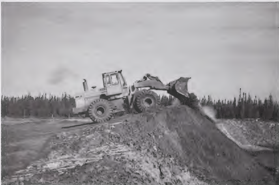
PHOTO 7-2. Co-filtered tailings being dumped on the ramp.
